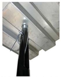
4. Raise the tool against the decking, rotate the Lagmaster™ pole tool until the collar of the I-LAG™ screw is flush with the decking.
