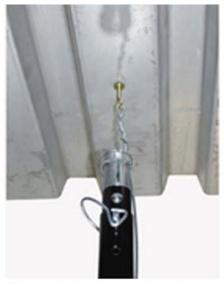
Rotate the Lagmaster<sup>™</sup> again to twist the wire, Lower the pole tool to complete the installation.
